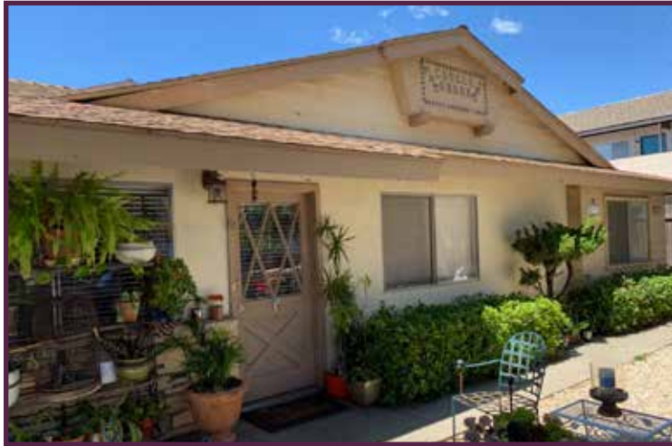
Front of Building
