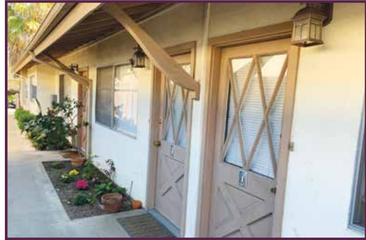
All Entry Doors on Ground Level
