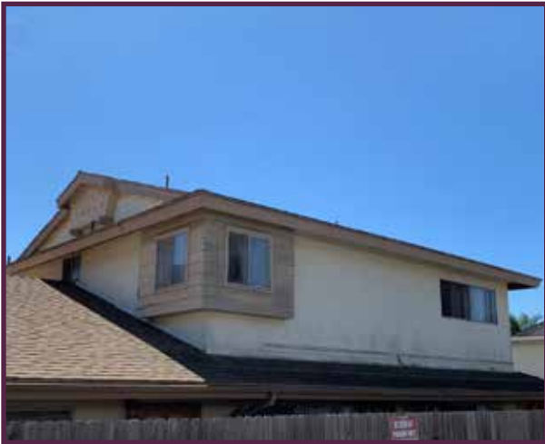
2nd Story - Upstairs of Units C & D
